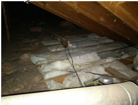
Vapor retarder/barrier installed wrong side up
