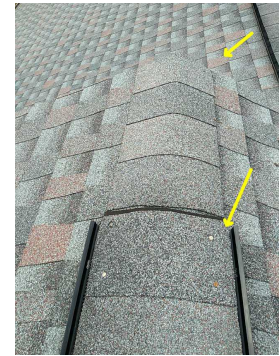
Exposed fasteners
