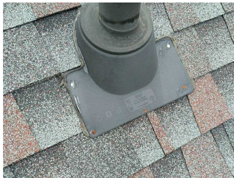
Exposed fasteners
